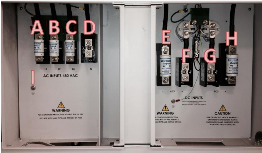
Figure 6: Wiring Compartment (Safety plexi-glass covers not shown in above figure for clarity)
